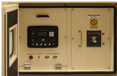
Control panel and breaker (rear side)
