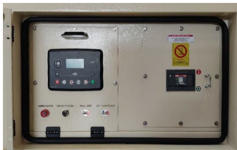
Control panel and breaker (rear side)
