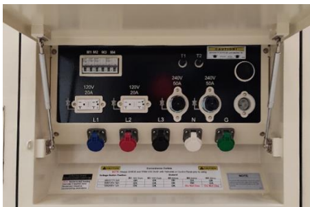
Connection Cam-Lock Standard
